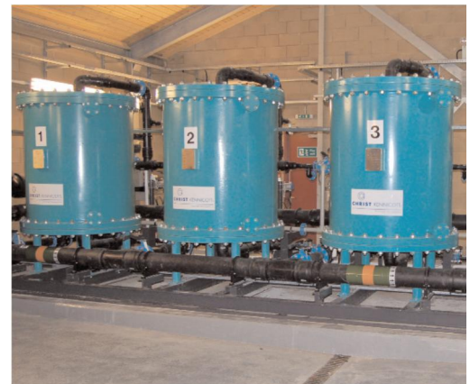
CENTRE. Skid-mounted filtration unit for installation at Severn Trent Water's Far Baulker site comprising Self-Cleaning BOLLFILTER Automatic with manual Simplex strainer as standby.
